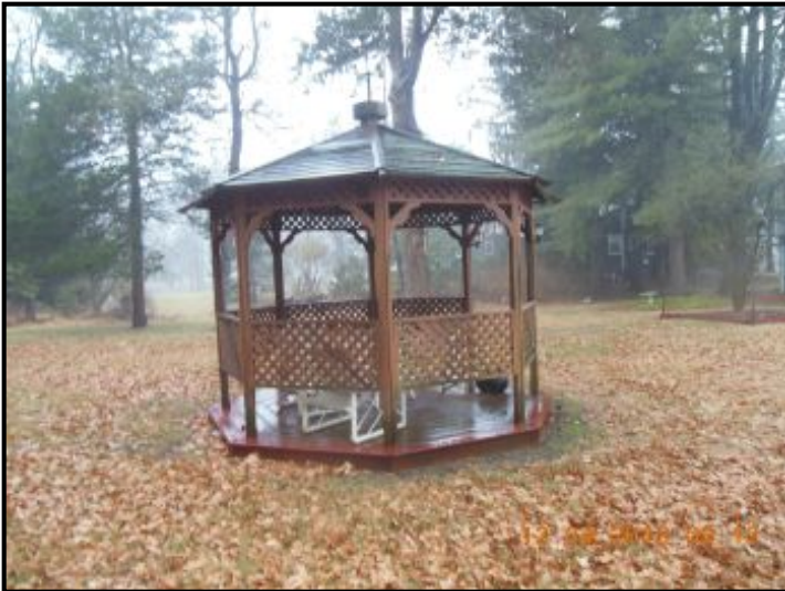
Detached gazebo in yard is in serviceable condition
