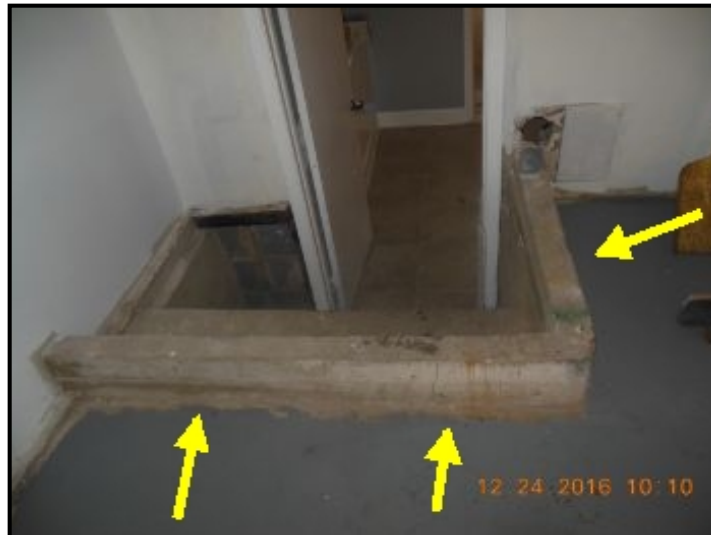
Bricks are installed around perimeter of stairwell in garage
