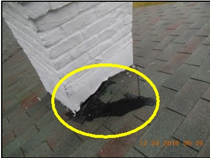
Roof cement repairs noted at cricket above the heating system chimney
