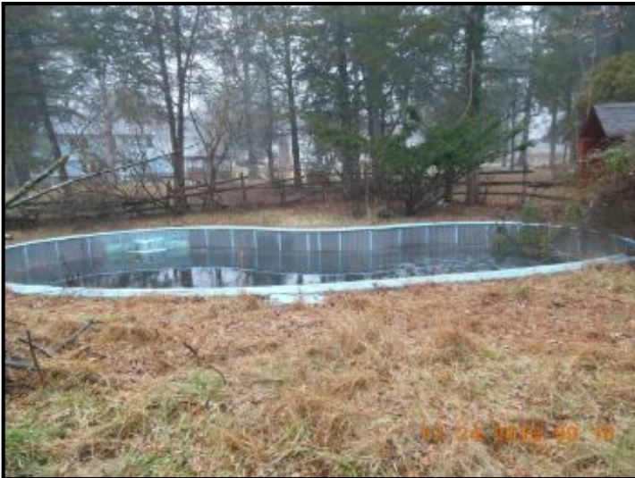
Underground pool is in poor condition
