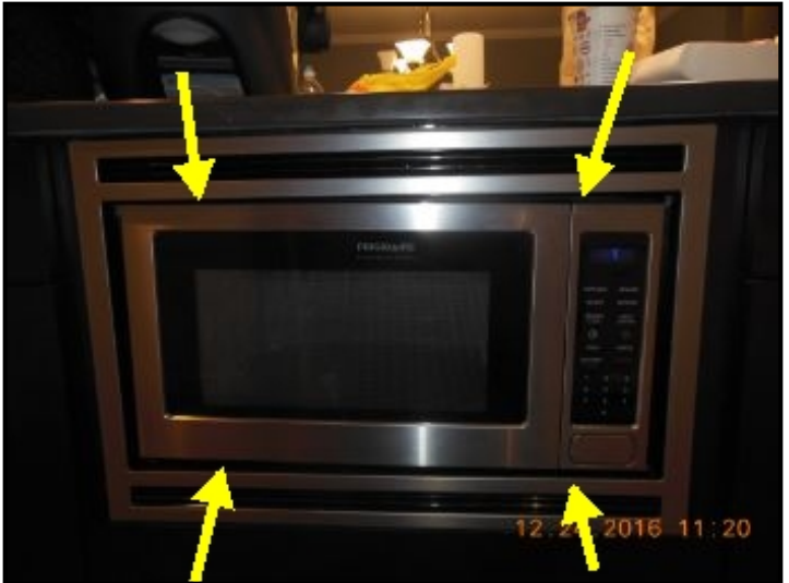
Trim piece around microwave oven is not installed properly Cabinet trim piece is installed unevenly and loose around microwave oven
