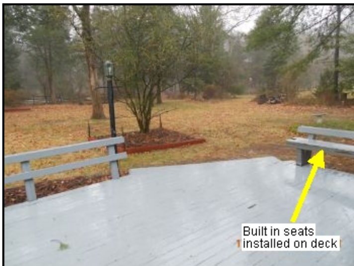
Built in seats noted on deck
