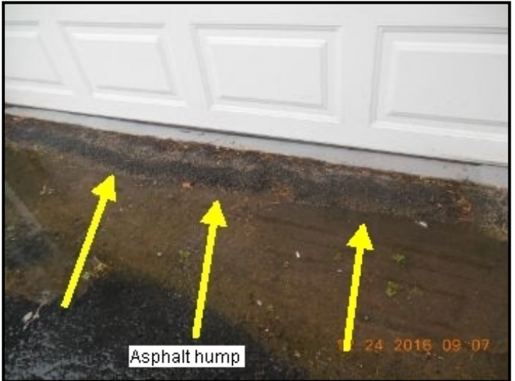
Water collects in front of garage vehicle door with hump of asphalt installed to prevent water leakage into the garage
