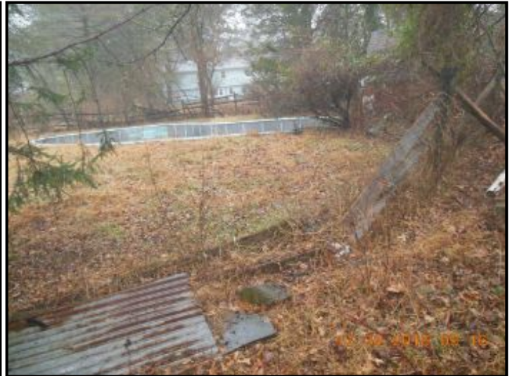
Fence around pool is collapsed
