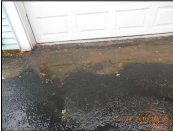
Water collects in front of garage vehicle door with hump of asphalt installed to prevent water leakage into the garage
