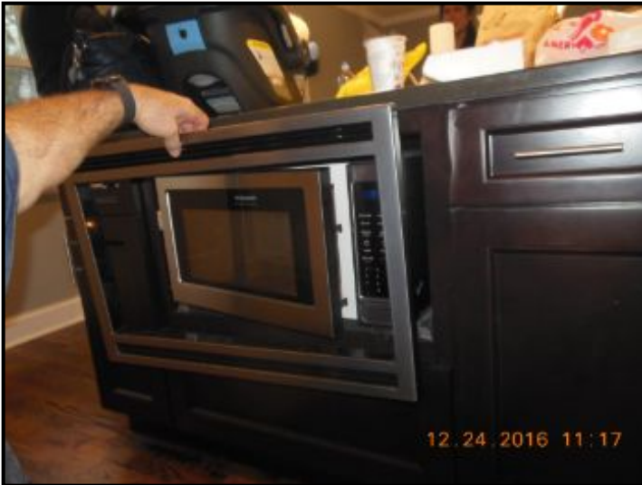
Trim piece around microwave oven is not installed properly Cabinet trim piece is installed unevenly and loose around microwave oven
