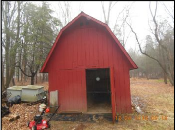
Shed installed in yard is in general good condition
